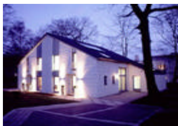
Figure 4: All the installations in inHaus are hidden behind walls and tiles (Source: http://www.inhaus-nrw.de )
